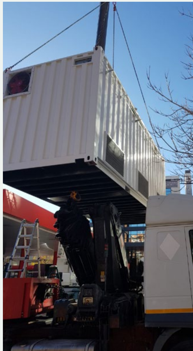
Installation of a hydrogen station in Madrid, Spain.
