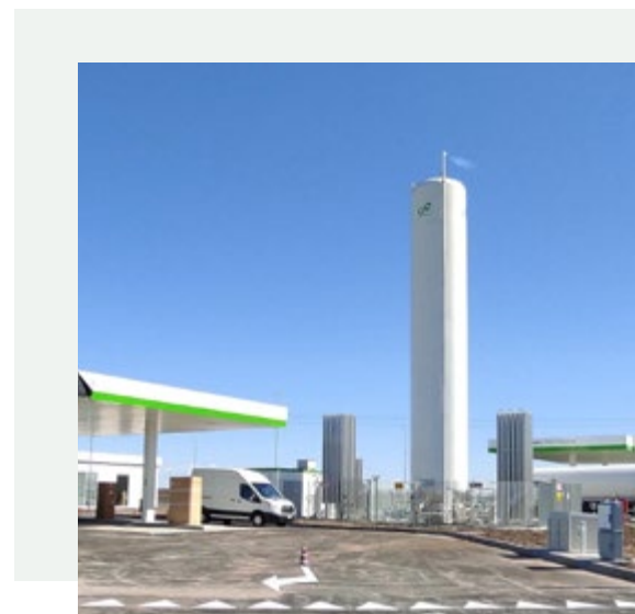
Multifuel station developed in Castel San Giovanni, Italy.
