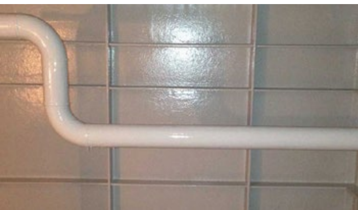
Refurbished tank for water storage.
