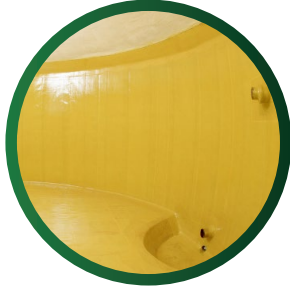
Epoflex® TW lining applied in a water storage tank.
