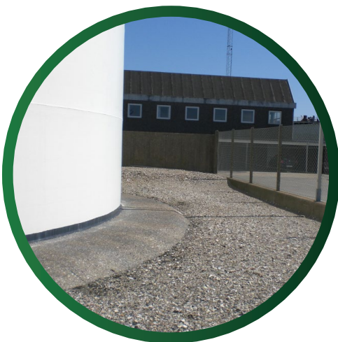
Restored ring wall of an aboveground storage tank.
