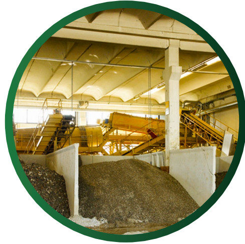
Wolf tank's soil washing plant with different types of soil separated.
