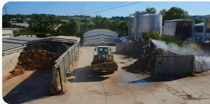
Recycling plant at Rovereta (Rimini, Italy).
