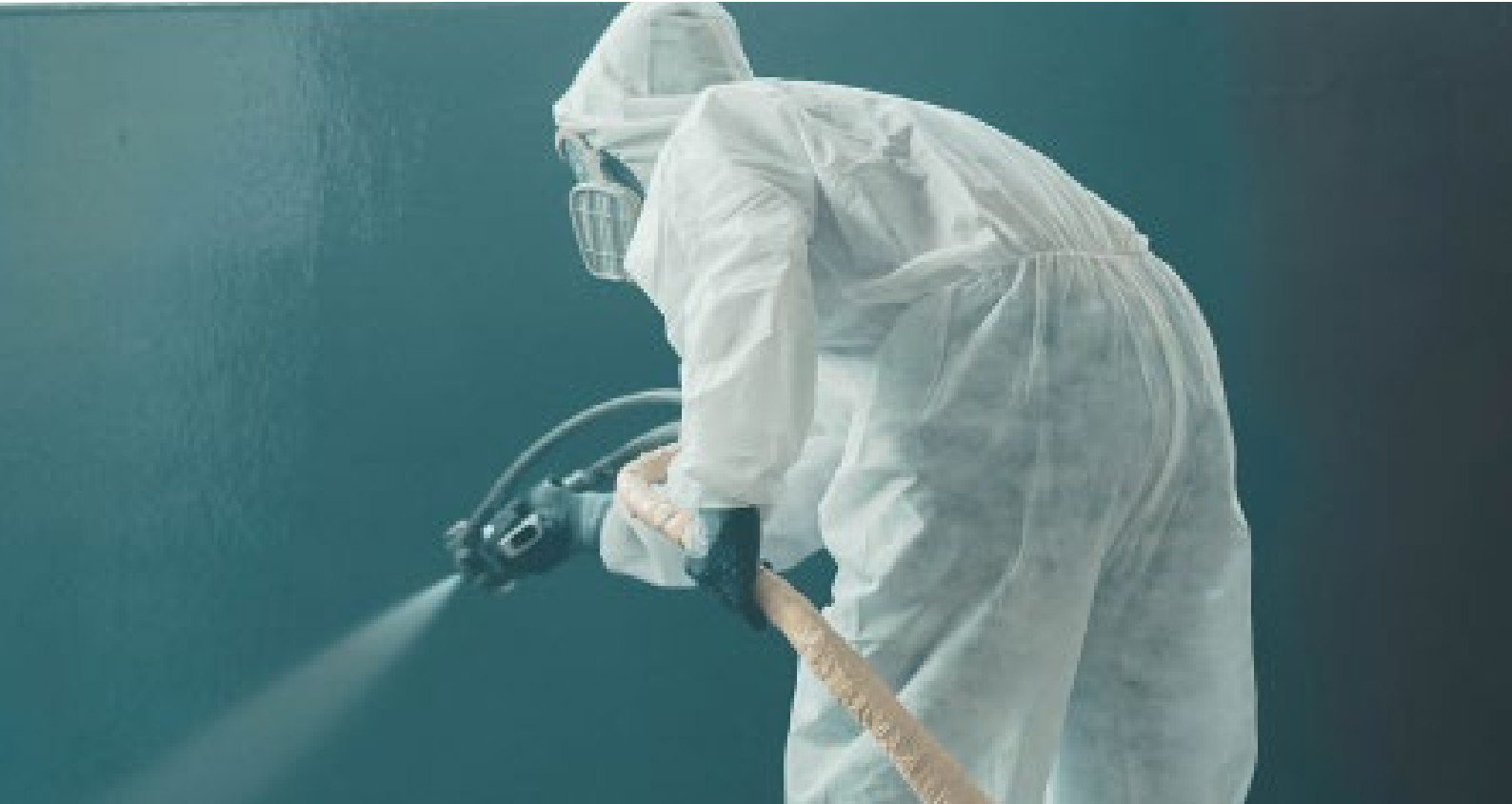
Aboveground tank coating application.
