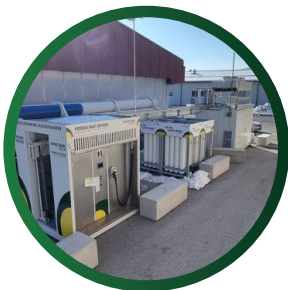
The Multi Hydrogen Fueling Station (MUHF) installed in Villach, Austria to refill local buses.
